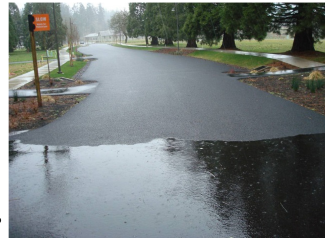
Porous asphalt next to standard asphalt.
