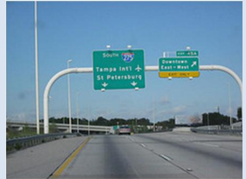
Potential FDOT signage structure
