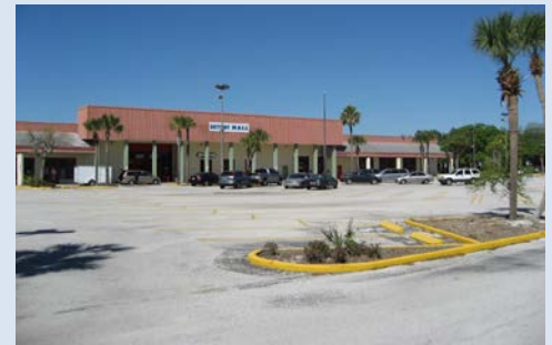
Skyway Mall Shopping Center
