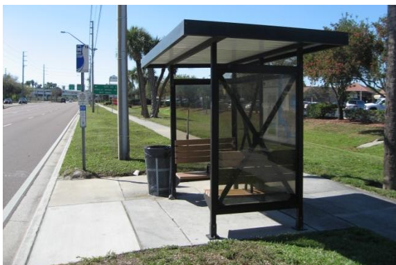
Current PSTA bus shelter
